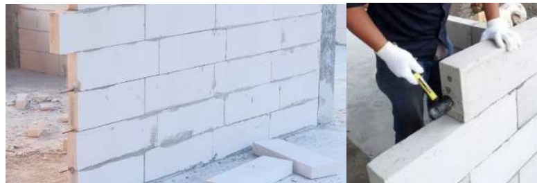
Gambar 5. 39 Material Dinding (Bata Ringan)
