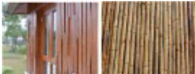
*Gambar 8.7 Dinding Bambu dan Papan Kayu*
