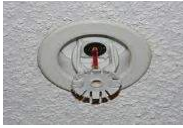
Gambar 5.16 splinker
