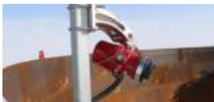
Gambar 5. 58 Flame detector
