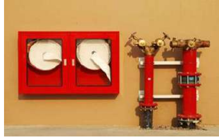
Gambar 5. 34. Hidrant gedung Sumber : https://firehydrant.id
