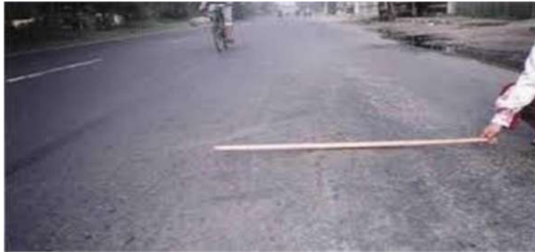
Gambar 2.14 Jembul ( upheaval )
