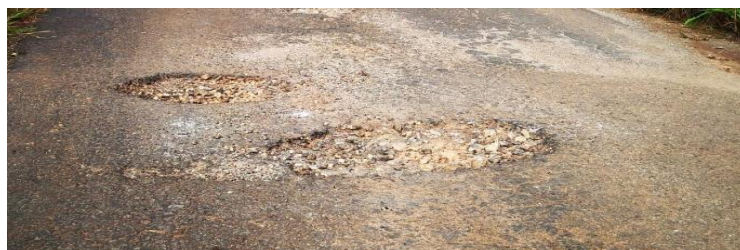
Gambar 2.5 Lubang ( Potholes )
