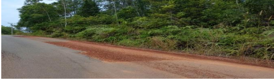
Gambar 2.4 Tambalan dan Tambalan Galian Utilitas ( Patching and Utility Cut Patching )
