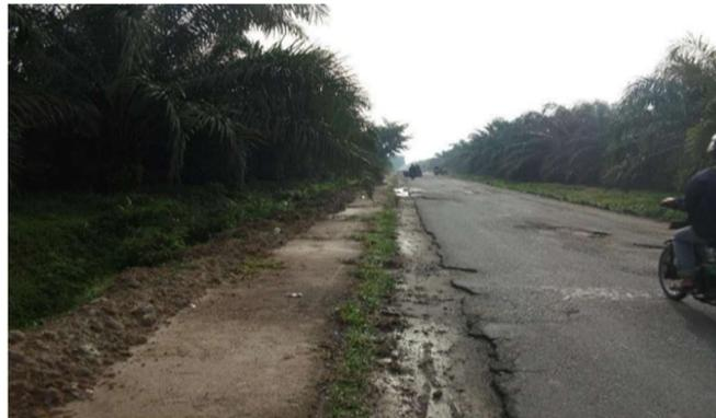
Gambar 2. 6 Cacat Tepi Perkerasan
