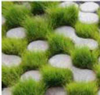
Gambar 4-0-8. Perkerasan grass block.
