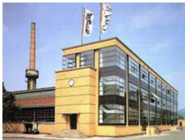
Gambar 2.3 Fagus Factory, Alfeld-an-der-Line, Walter Gropius Sumber: (Guide To Modern Architecture, Rayner Banham)
