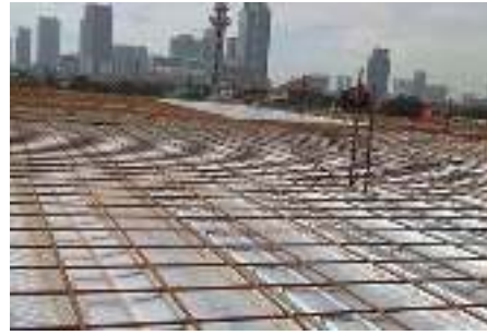
Gambar 72. Upper Structure Berupa Dak Beton
